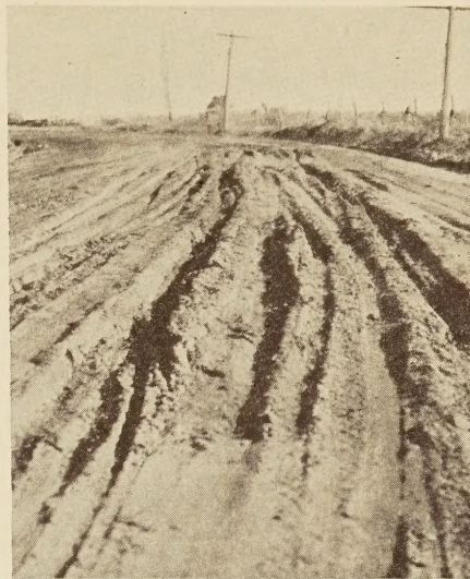
SURFACE DEEPLY RUTTED
